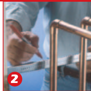
2 Position bracket and mark pipe locations
