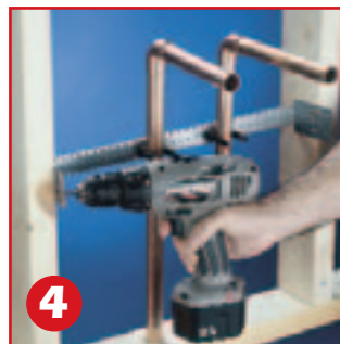
4 Install the TSGB to wall studs
