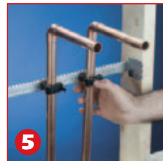
5 Secure the pipe by attaching TPC retainer
