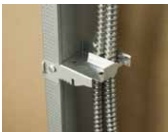
Metal Stud with MC/AC Cable
