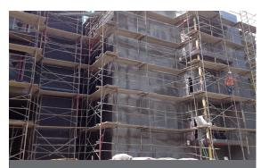
WNC relies upon heavy plastic and stucco tapes to protect surfaces as plaster is messy and can cause damage.
