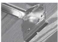
Two barbs on each side of brace will hold brace into position. Secure brace into wood with four, # 12-14 X 1" long lag screws.
